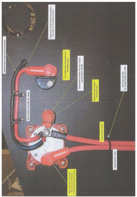
Standard Battery Switch Circuitry-Rear View
